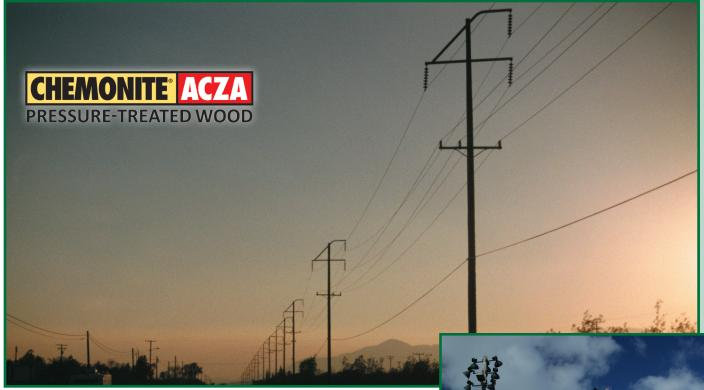
Chemonite® poles provide reliable transmission and distribution of electric energy, with practical benefits and less environmental impact than alternatives. The ACZA treatment consistently meets recognized standards of penetration and retention in difficult-to-treat species such as Douglas fir. Poles ranging from 25′ to 135′ are readily available from Conrad Forest Products.
